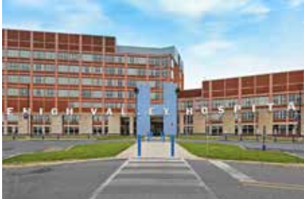
LVHN Cancer Center at Lehigh Valley Hospital-Muhlenberg
